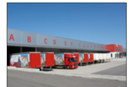
Teningen logistics centre
