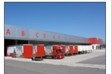
Teningen logistics centre
