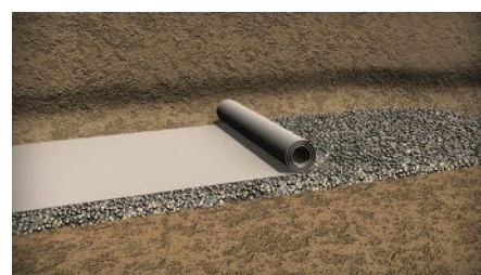
Figure 8: Laying geotextile
