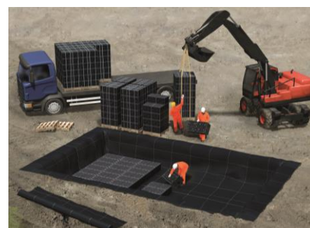
Figure 9: Positioning the infiltration ditch elements
