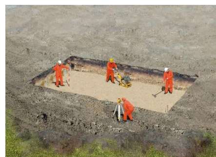
Figure 7: Preparation of the levelled ground
