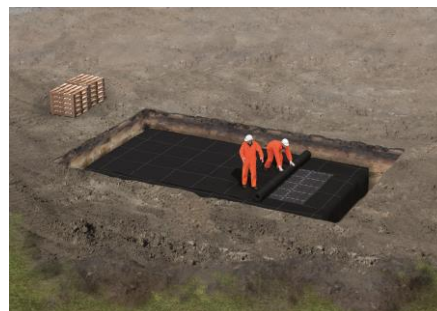
Figure 13: Wrapping with geotextile
