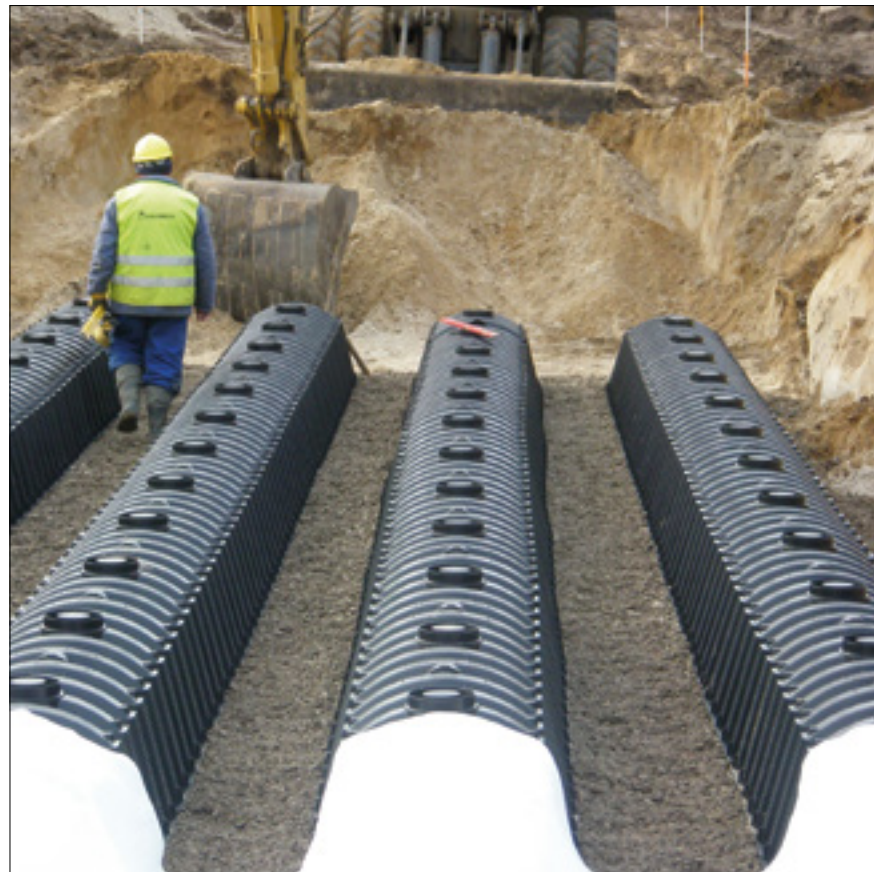
Industrial warehouse, Raben (PL)
