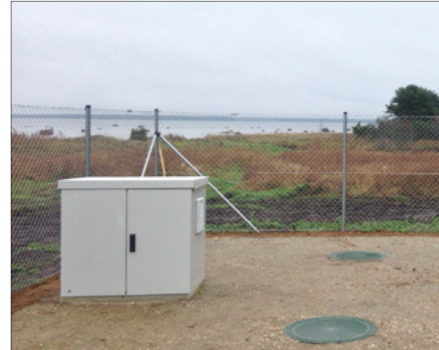
The image shows the External steel cabinet XL for 50 inhabitants
