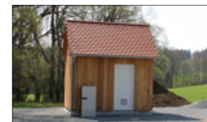
Example: Installation in a machine house
