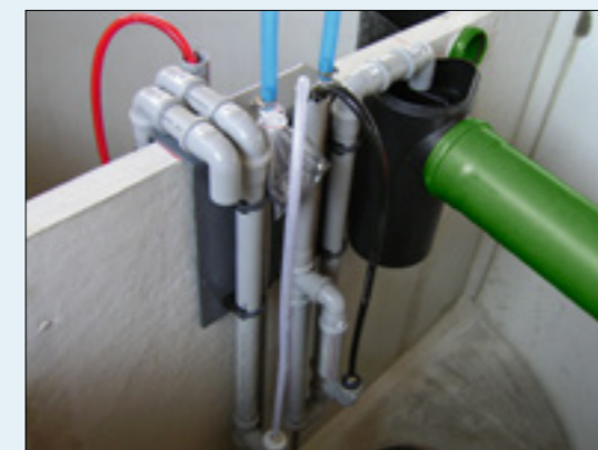
Image shows System pack for retrofitting > 28 inhabitants)
