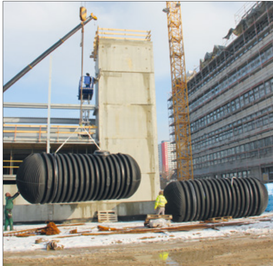
Industrial building, Neu-Isenburg (Germany)
