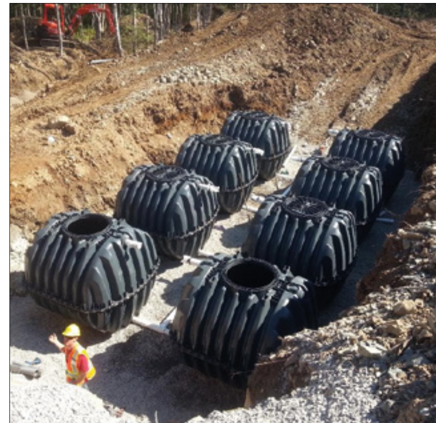
Industrial building, Nova Scotia (Canada)
